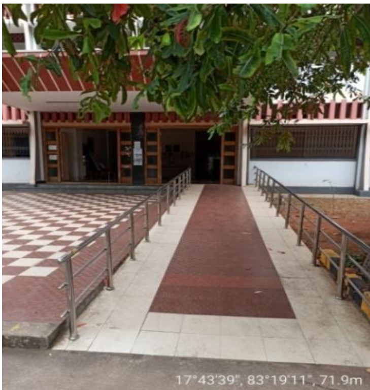
APPROACH RAMP FOR DISABLED AT CIVIL ENGINEERING CLASS ROOM COMPLEX
