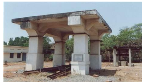
1000 KN Loading Frame
